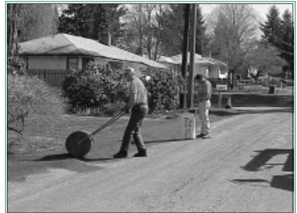
City workers construct some shoulder work to facilitate better drainage in Linwood.
